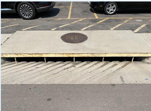
Typical Type-R (14) curb inlet with centered manhole
