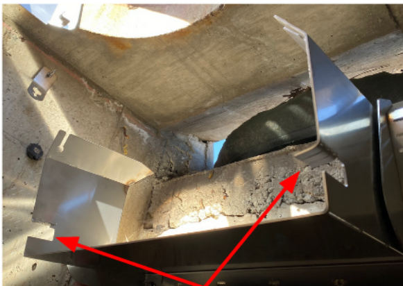
Three fingers on either side of Interface Funnel bent inward 90d
