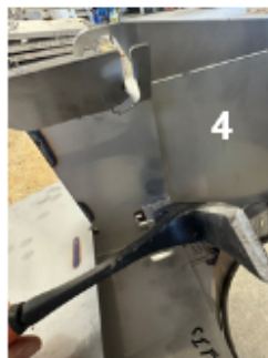
4. Hammer down finger(s) to lock in thumb
