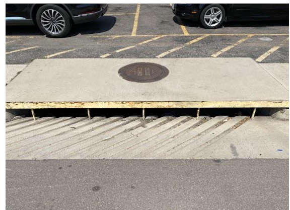
typical Type-R (14) curb inlet with centered manhole
